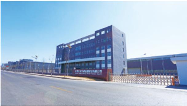
The building infrastructure of the Taiyuan processing centre was substantially completed and is under trial run currently. Equipped with coil and plate cutting, precision shearing and slitting, surface polishing and forming platforms, Taiyuan processing centre will provide processing services to both our stainless steel and carbon steel customers.
